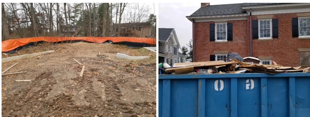
Pictured above are photos of the inadequately sized mark out and curbing for the trash and recycling containers onsite and construction waste container containing mandated materials mixed with trash.
